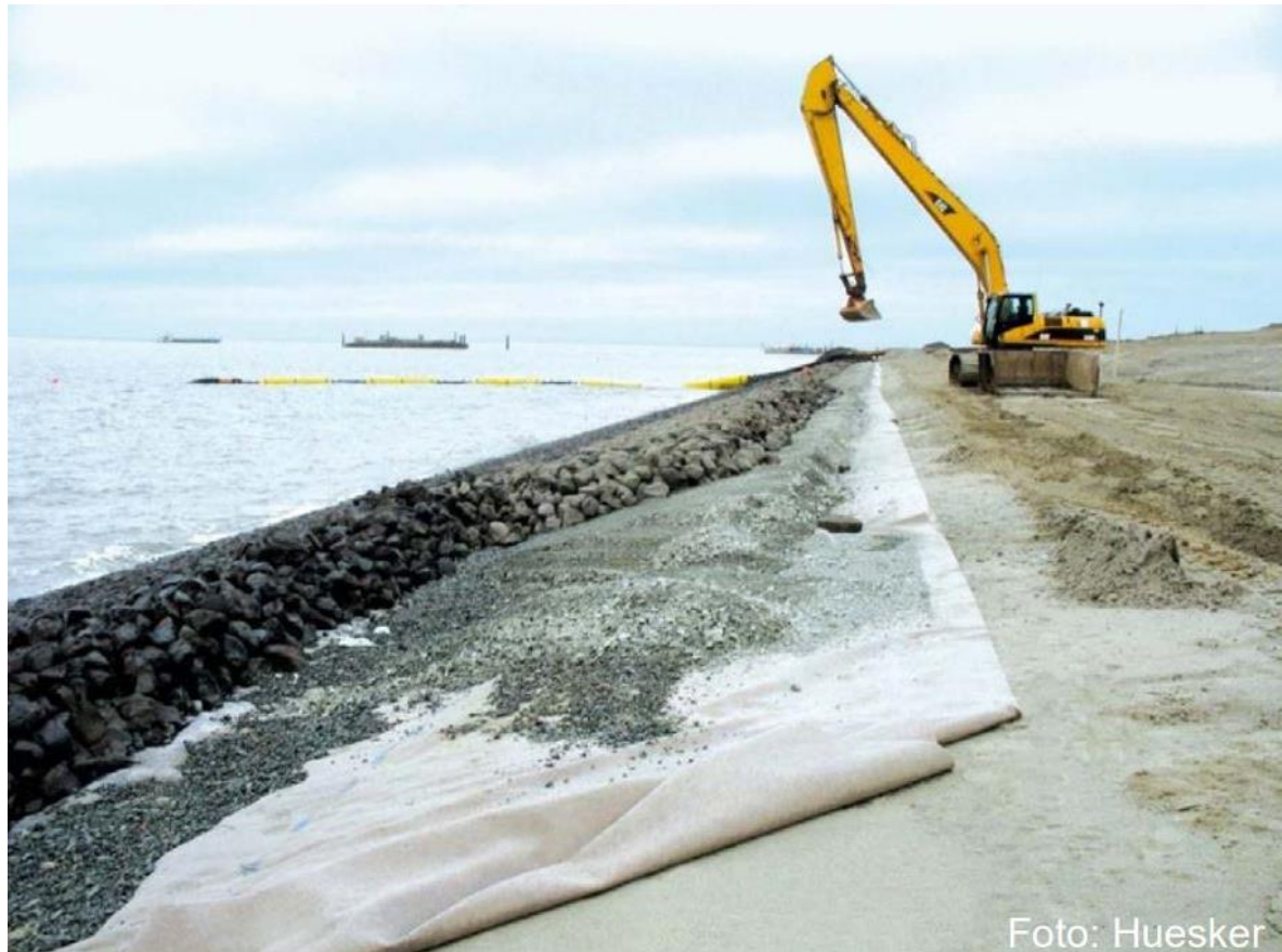
Figure 3. Installation of geotextile in a hydraulic application.
